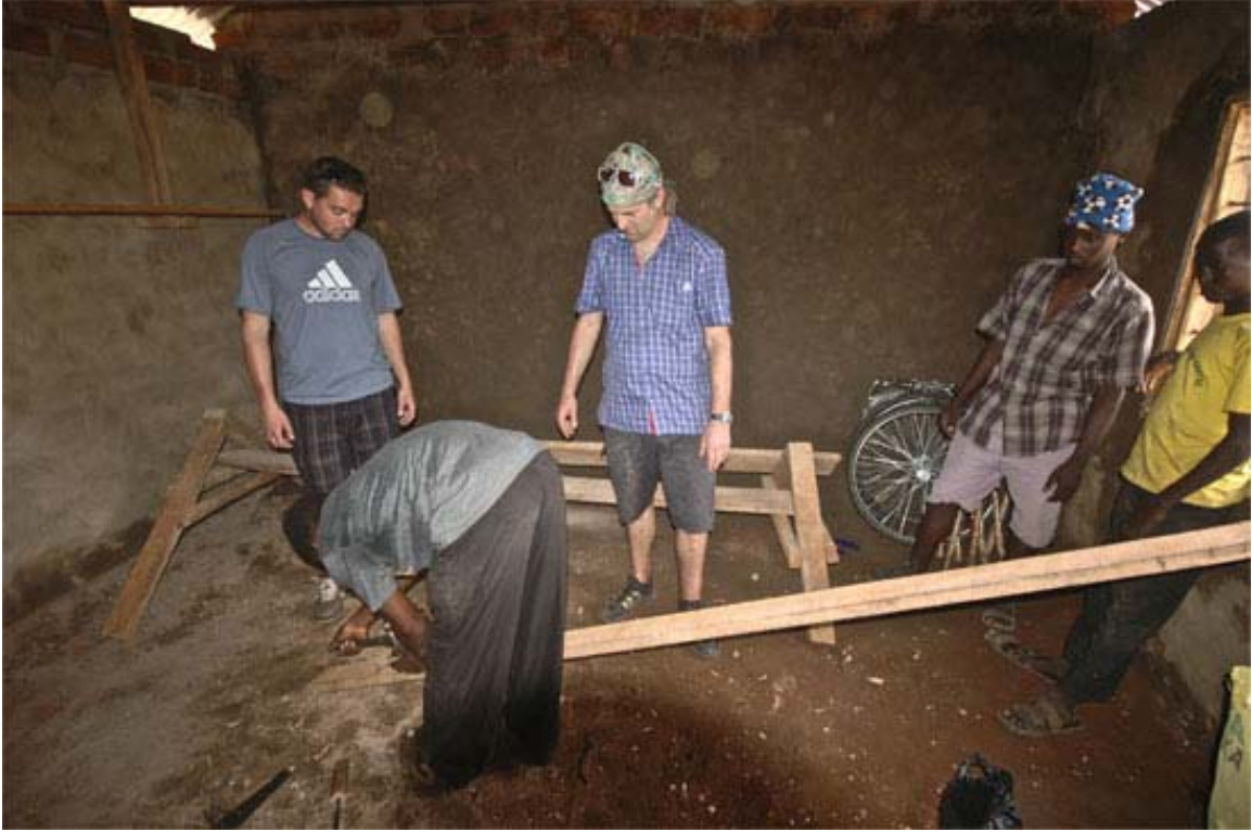
Our new shop under construction, with the help of the locals.
